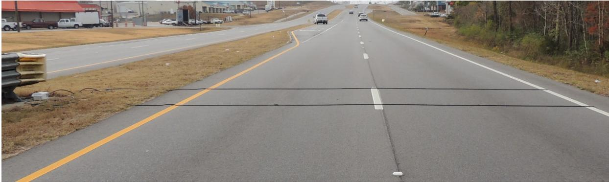
**Figure A1. Example of road tubes installation.**
